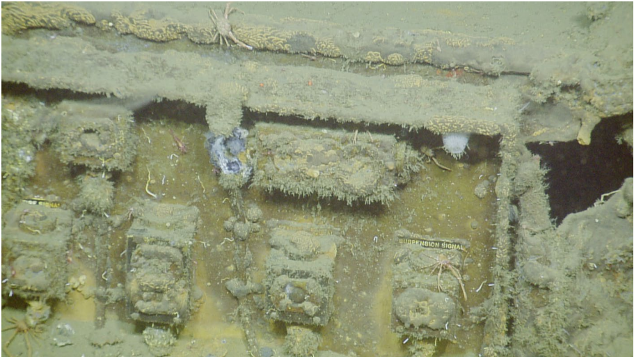
Fig. 10 ROV image of switch panel on the navigation level with plastic labels still readable. Image courtesy of Ocean Exploration Trust
