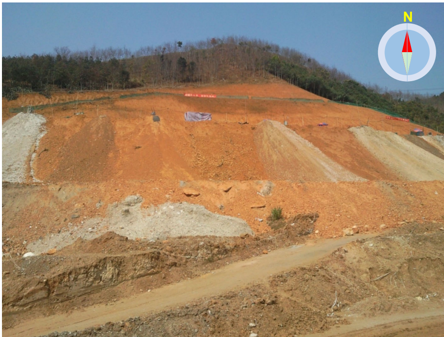
Fig. 19 The soft rock highway slope located in southern China
