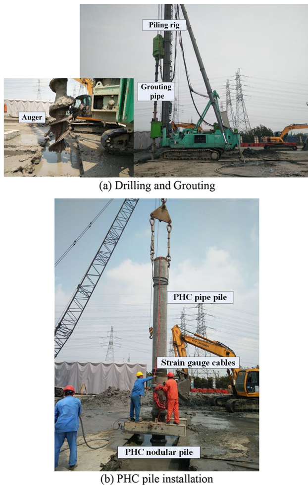
Fig. 4 PGP pile installation process
