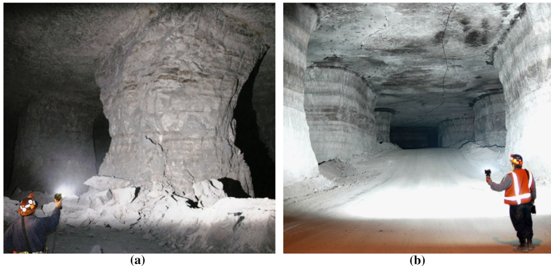
Fig. 14 Failure modes of underground rock pillars observed by Esterhuizen et al. [8]: a Typical hourglass shaped pillar; b Pillars at deeper stone mines
