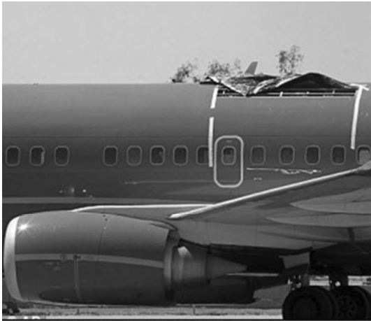
Figure 2 Tarpaulin covering the five-foot-hole that ripped open roof, from ref. [12].
