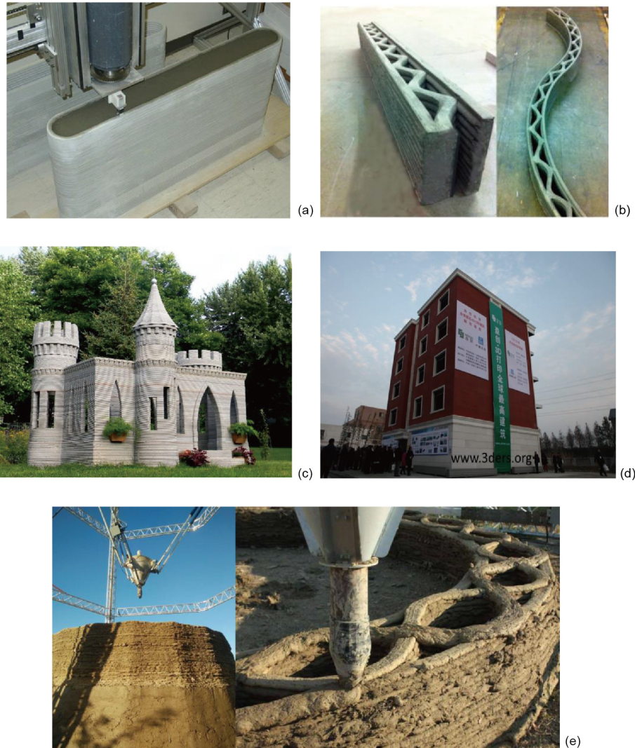
Figure 5 (Color online) Examples of full scale builds from contour crafting printing. (a) Concrete wall with a height of 60 cm; (b) hollow walls with corrugated internal structure; (c) castle printed in-situ ; (d) five-story apartment built by WinSun; (e) clay and straw wall, over 2 m and still growing.
