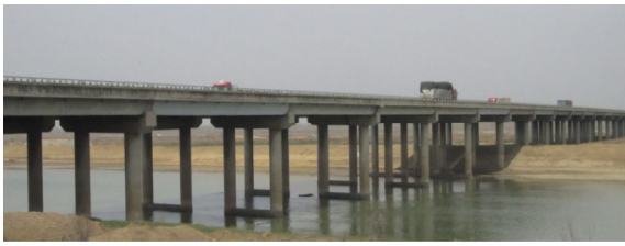
Figure 12 (Color online) Overall view of Xinyihe Bridge.
