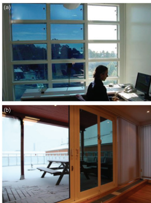
Figure 1 Two examples of multi-panes of EC smart windows [8]. (a) An application of EC smart windows produced by Sage Electrochromics in an office at the Lawrence Berkeley National Laboratory, USA; (b) an application of EC smart windows produced by ChromoGenics AB in the company's premises in Uppsala, Sweden (color online).
