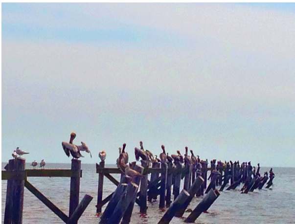
Fig. 2 Pelicans on a broken pier, Gulf of Mexico (Luther ©2014)
