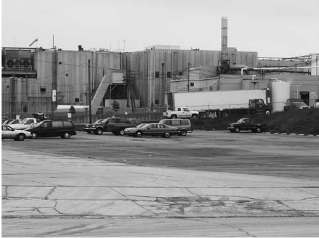
Photo 1 A view of the plant taken on May 1, 2006, the “Day Without Immigrants.” Note the near-empty parking lot
