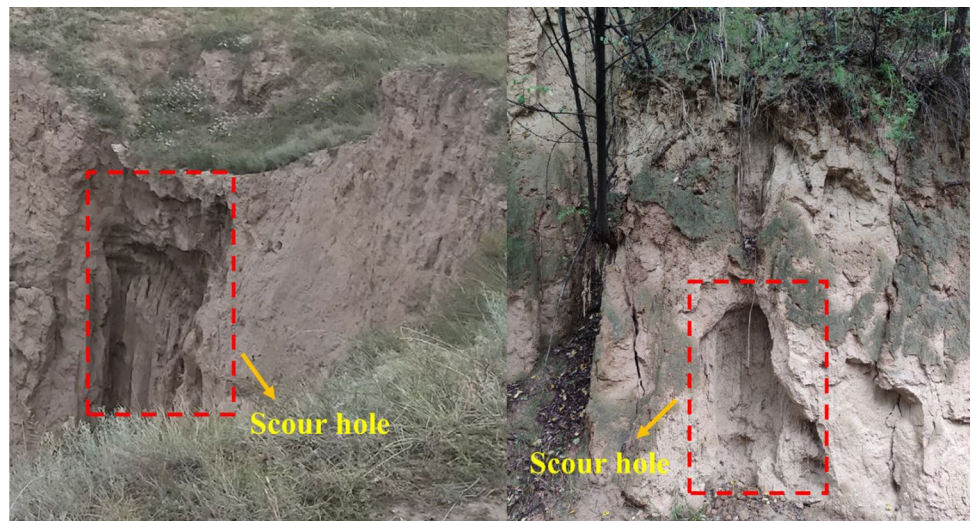
Fig. 11 Morphological characteristics of scour holes in gully headwalls
