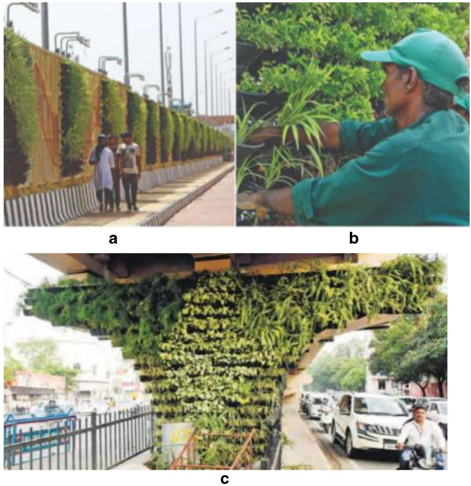
Fig. 13 A and B Nizamuddin Bridge, Delhi (DNA n.d.); C Begumpet Flyover, Hyderabad (Express n.d.)
