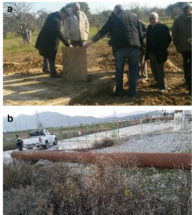
Fig. 7 a,b Laying pipes in agricultural areas
