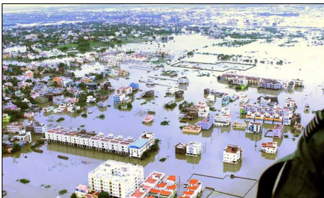
Fig. 4 Chennai floods 2015 (view of Chennai submerged in storm water flood)
