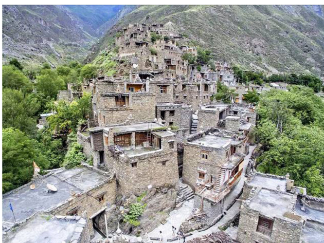
Fig. 4 Masonry building complex
