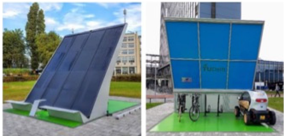
Fig. 2 Front and back view of solar e-bike charging station. Retrieved from (Chandra Mouli et al. 2020)
