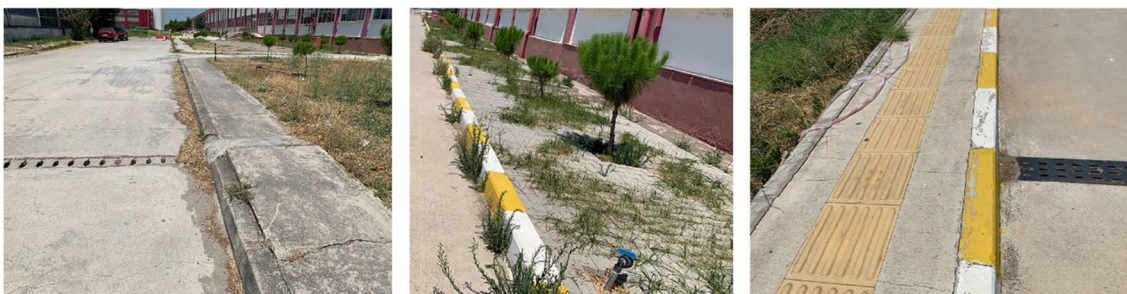
Fig. 10 Pavement paving materials
