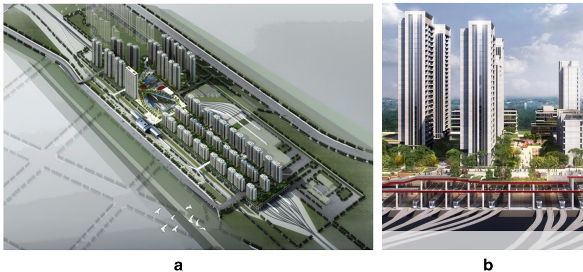
Fig. 3 Renderings of the over-track buildings on top of the metro depot. a Full view, b cross-section profile
