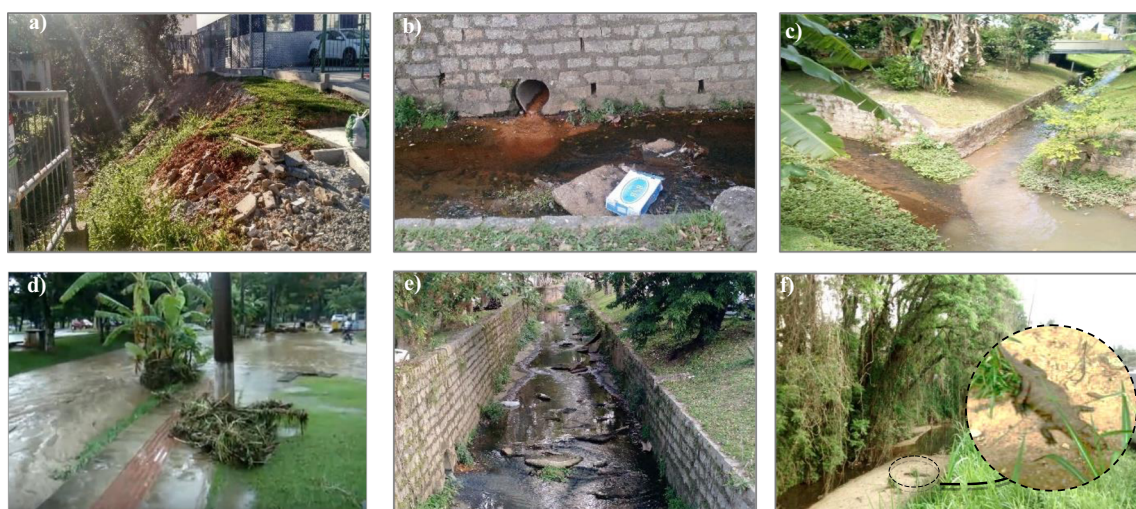
Fig. 6 a Public works outside the UFSC and construction waste on the Eletrosul riverbank. b Construction waste (sediments) arriving at UFSC. c The confluence of Três Córregos and Serrinha rivers. d Três Córregos River flood (inside UFSC). e Usual flow of rivers, where it is observed
