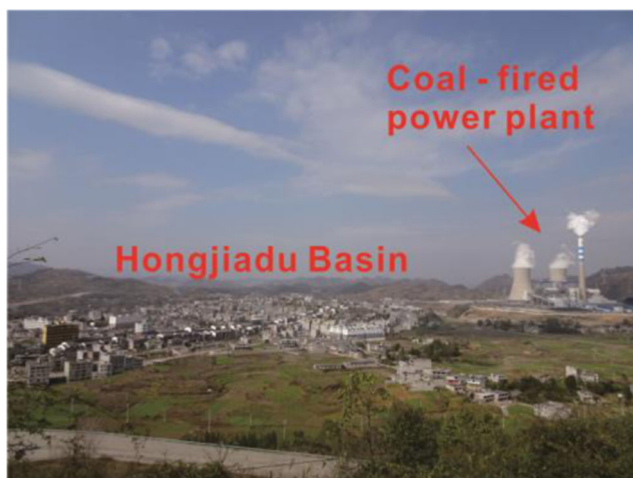
Fig. 7 A large coal-fired power plant located in the Hongjiadu Basin
