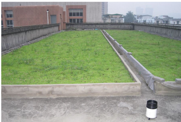
Fig. 3 Photograph of Green Roof A (in left) and Green Roof B (in right) during the monitoring period
