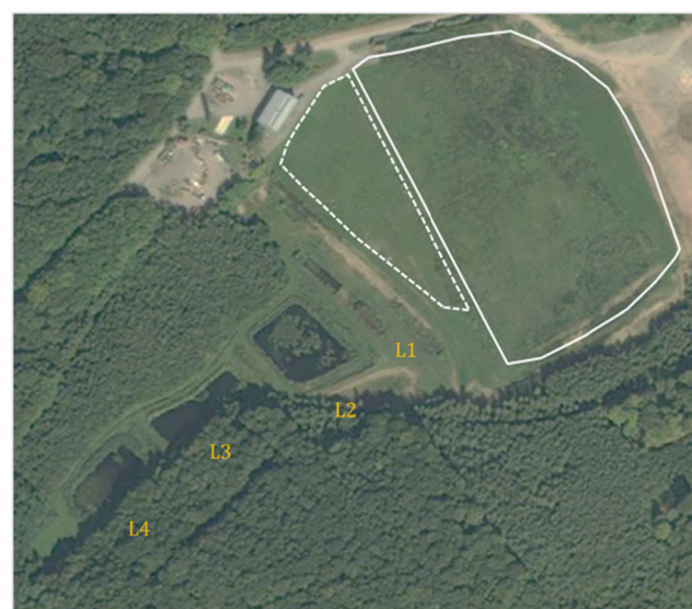
Fig. 1 The Etueffont landfill with lagooning ponds (L1: sampling pond, L2, L3 and L4) and location of old landfill (OL) and new cell leachates (NC) (top). Aerial view of the landfill (bottom)
