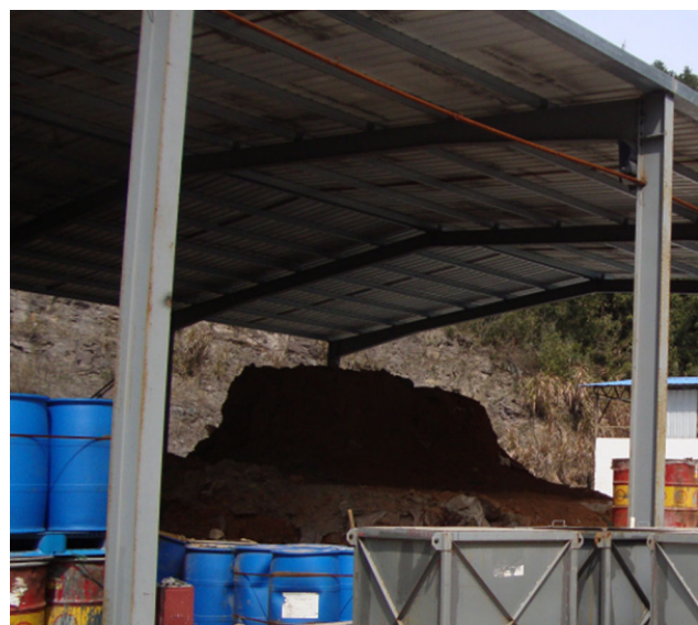
Fig. 2 Covered depot of contaminated soil
