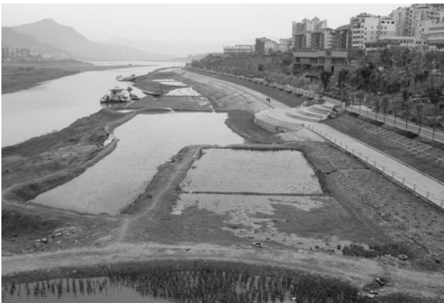
Fig. 5 The photograph taken 16 April 2012 shows some of the engineering of the banks of Hanfeng Lake which is a distinct part of the Three Gorges Reservoir lying within Kai City in Kaixian, a county-level administrative unit in Chongqing Municipality, China. The lake level had been lowered following its winter peak to reveal artificially created dike ponds which were designed to maintain desirable aquatic plants at the water’s edge throughout the fluctuation cycle of the lake level. Hardened sloping surfaces and lakeside recreational amenities are also visible
