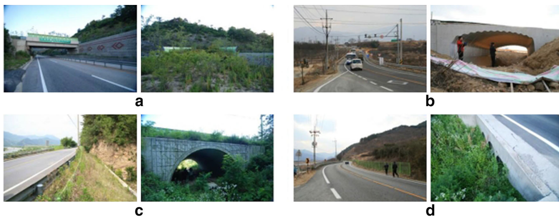
Fig. 6 Four wildlife crossings constructed as a result of this study: a Overpass 1 crosses from hill to hill where a mammal roadkill hotspot occurred on local road 19. b Underpass 1, located across the edge of agricultural land and mountains, is under construction. c Underpass 2 is a crossing on the riverside road that links the upland,
