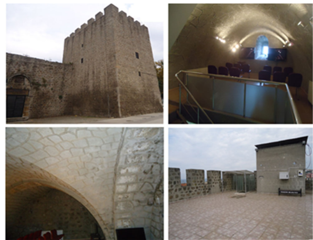
Fig. 1 Pictures of Zağanos Bastion
