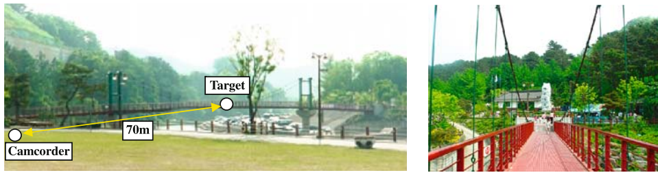
Fig. 8. A pedestrian suspension bridge
