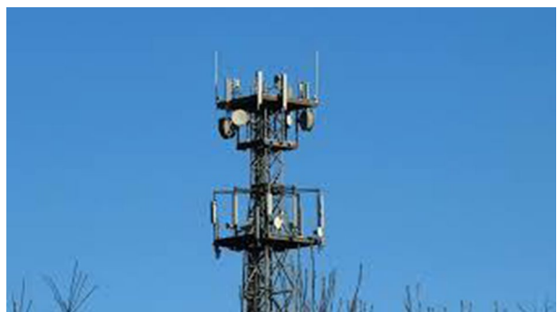
Fig. 5 Network Installation in open area for coverage settings
