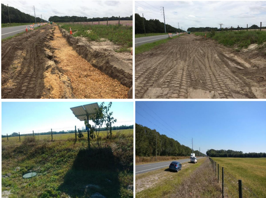
Fig. 1 Schematic flowchart for design, construction, and operation strategy in the field including construction phase (upper left); completion of construction of B&G media section (upper right);
