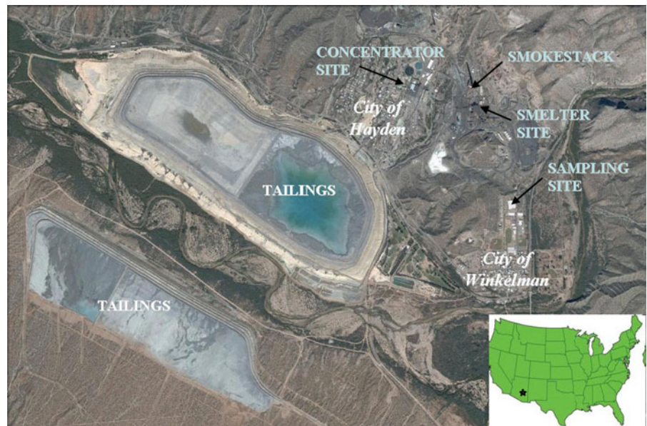
Fig. 1 Satellite map of Hayden/Winkelman, AZ, with locations of mining and sampling operations. Top of the map is North and size of map is approximately 4.3 km by 6.6 km. The smokestack is 305 m tall. Terrain topography around the shown area is complex: elevation increases towards the North with a narrow valley extending in the NW–SE direction. Source: Google Maps
