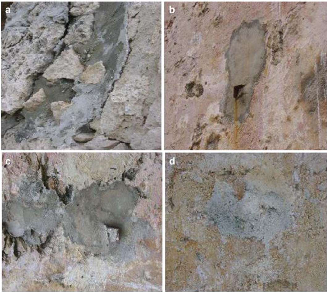
Fig. 12 a–d Use of Portland cement mortar at San Carlos fortress
