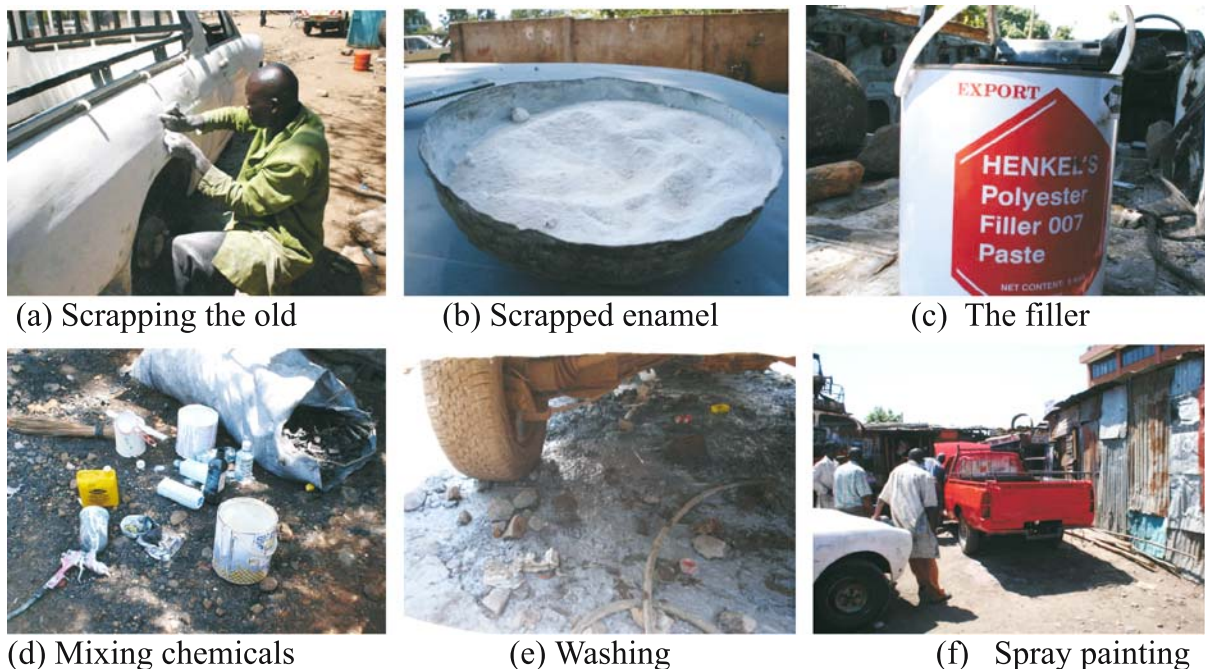
Fig. 5 The spray painting process and wastes
