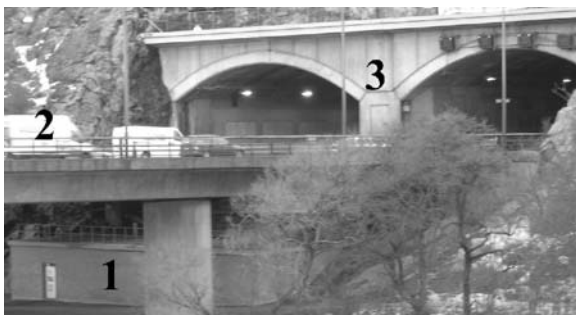
Figure 2 The treatment plant for road runoff (1) is located under a bridge (2) (cf. Figure 1). The southern entrance of the Fredhäll tunnel is visible (3).
