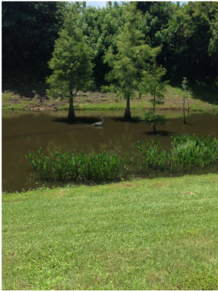
(a) Constructed wetland
