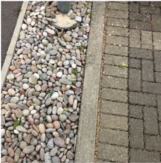
(k) Infiltration trench
