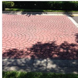
(n) Porous pavement
