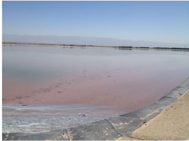
Fig. 8 Reddish brown scum layer in the anaerobic lagoon
