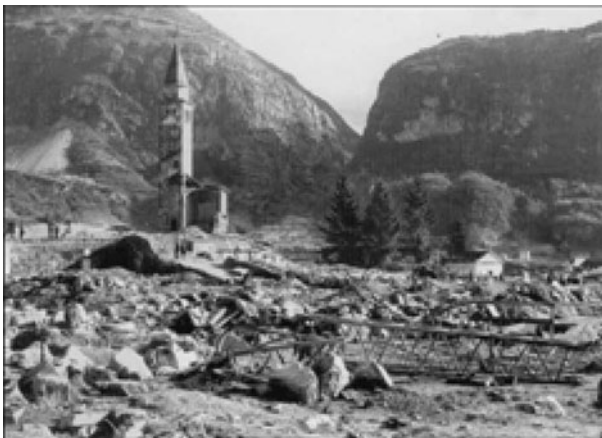
Fig. 10 Pirago's bell tower: the only building left standing in the village after the transit of the wave (Zanfron 2006)
