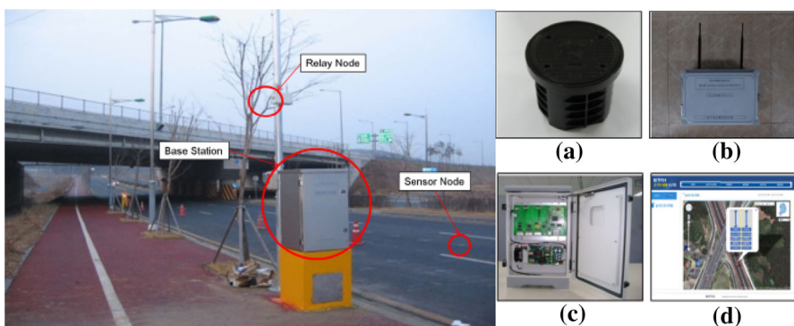
Fig. 6 Photographs of our testbed: a a sensor node, b relay node, c base station, and d monitoring server
