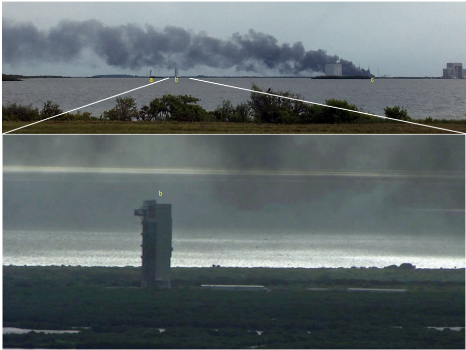
Fig. 28 The launch pad (a) at Space Launch Complex 41 with the VIF (b) with OSIRIS-REx inside is seen through the smoke from the AMOS-6/SpaceX Falcon 9 static fire test explosion and fire at the adjacent Space Launch Complex 40 (c) on September 1, 2016. Although the VIF was only about 2 km downwind from the fire and the shared water pump between the launch sites was damaged, OSIRIS-REx was protected from contamination due to a combination of planning and swift work. Photo credit: Top : Dworkin, Bottom : (Clark 2016b)
