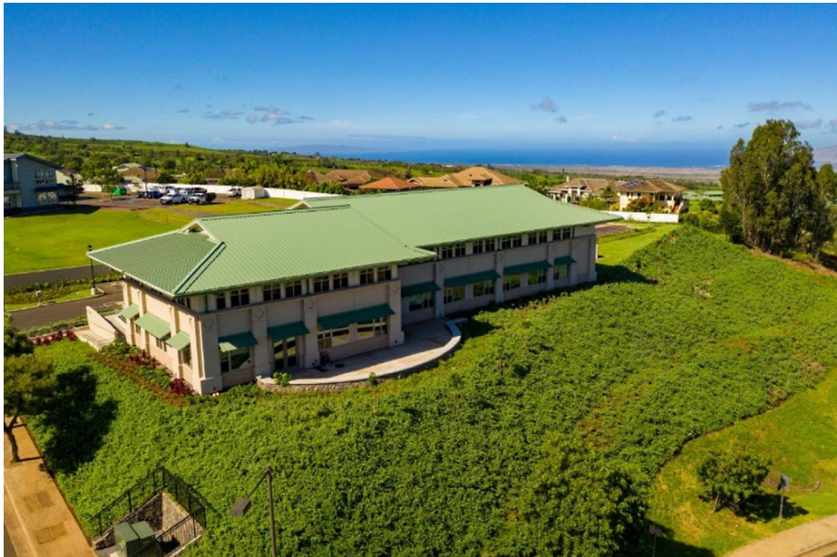
Figure 14 The DKIST Science Support Center (DSSC) in Pukalani, Maui, Hawai'i. This base facility provides office and lab space and includes a remote operations room from which observations can be monitored and guided by science staff.
