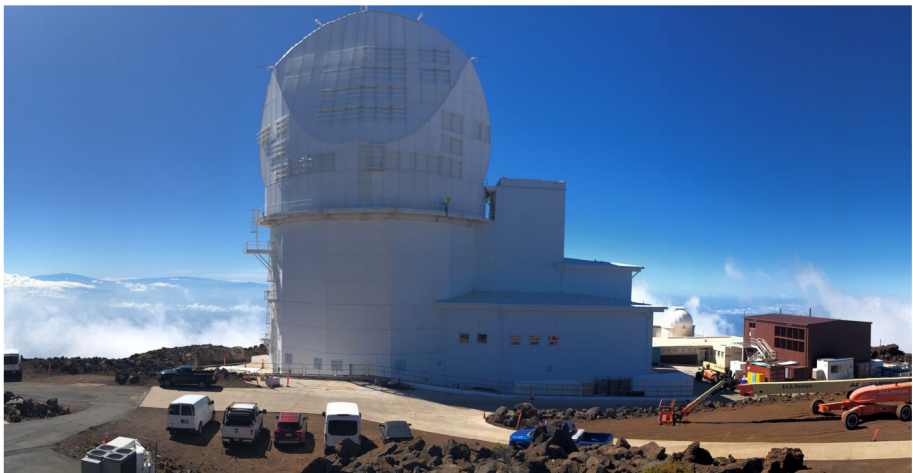
Figure 2 The outside of the completed DKIST on Haleakalā. The telescope building with lower and upper enclosure and the attached Support and Operations building, including platform lift used to transport M1 to the telescope level, are shown on the right of the image. Vent gates ensure sufficient air flow through the enclosure during operations. The utility building, which supplies coolant to the main facility and houses backup power systems is visible to the right of the main facility. The overall facility height is 41.4 m.
