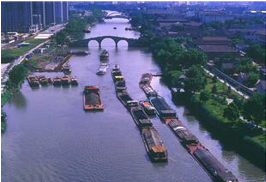
Fig. 2 Construction of the Grand Canal from Hangzhou to Beijing began during the Qin Dynasty, in 219 B.C. This canal was the primary canal for water traffic in China until recently, and now forms the eastern branch of China's South to North Water Transfer Project. Source: http://lvyoubaidu.com/jinghangdayunhehangzhouduan
