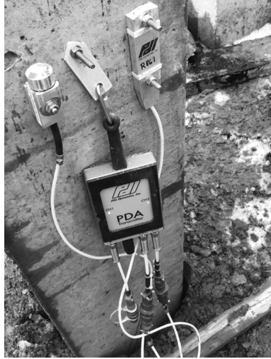
Fig. 1. A driven pile with sensors installed for testing by the wave theory of impact.
