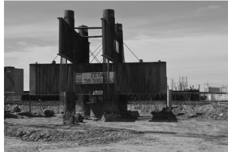
Fig. 1. Vertical static pile tests using the SCQLT method.
