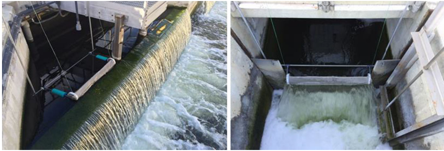
Fig. 4 A surface filtering assembly used for collecting microplastics-containing wastewater system (Carr et al. 2016)
