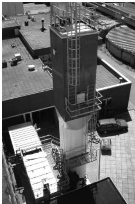
Figure 3. Anammox reactor at Rotterdam WWTP (Courtesy Paques and ZHEW) in EU-icoN project.
