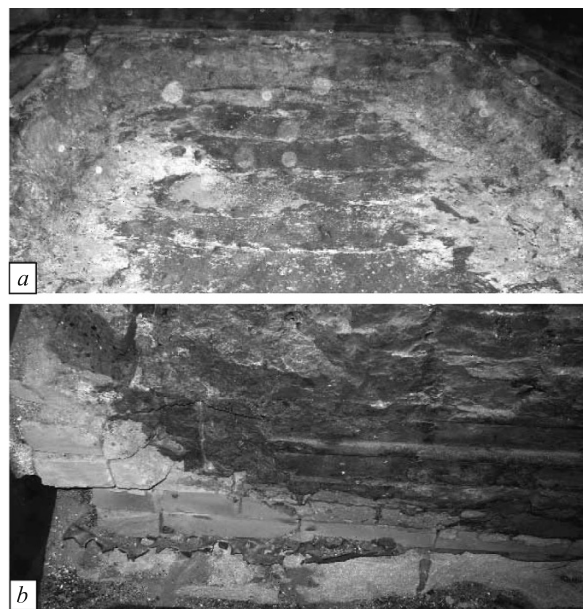
Fig. 1. Hearth surface condition constructed from graphitized blocks with 70–80% graphite (a); b) block cross section.
