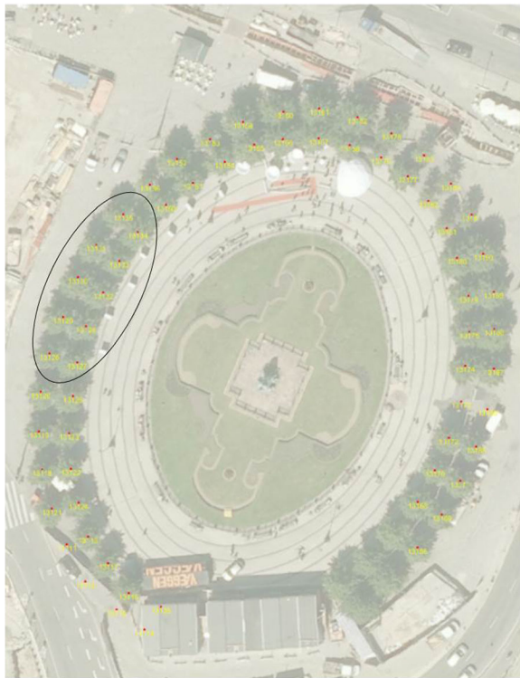
Fig. 1 Aerial picture of the tree planting at Kongens Nytorv. The two ellipses of trees are planted in connected structural soil bands. Test trees are encircled. Picture supplied by the Municipality of Copenhagen
