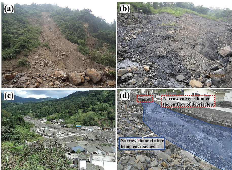
Fig. 3 The occurrence of debris flow in the Niutang Gully. (a) Debris flow source generated by collapse. (b) Debris flow source generated by landslides. (c) The water treatment plant was inundated by the 8.20 debris flow. (d) Encroachment of buildings upon the debris flow channel
