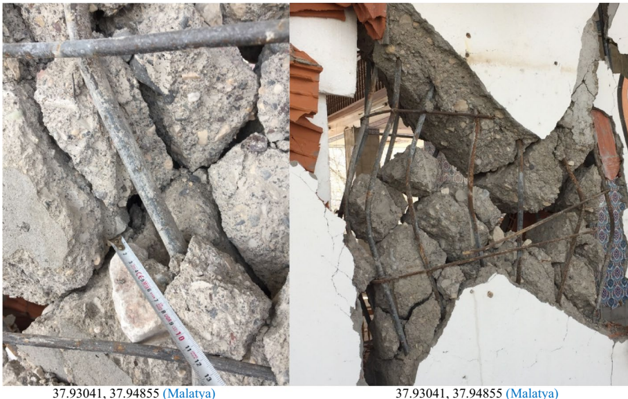
Fig. 24 Material quality of old buildings
