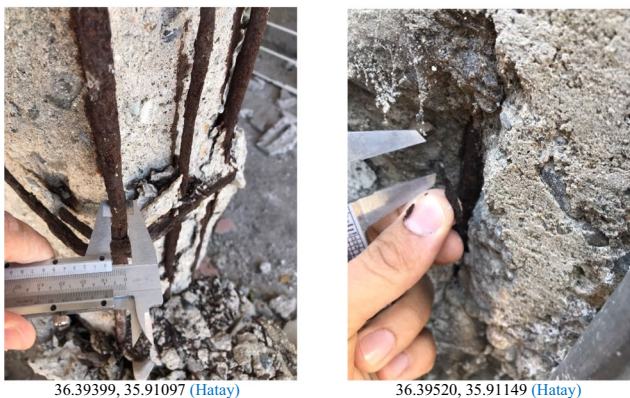
Fig. 28 Corroded reinforcement
