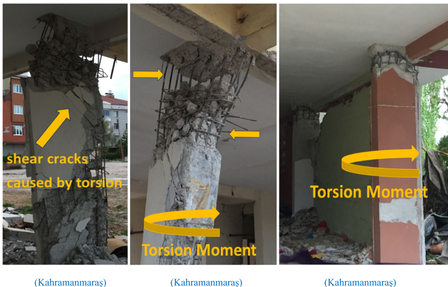
Fig. 23 Torsion damage
