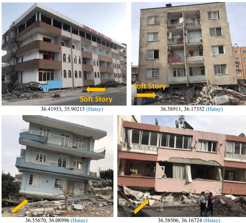
Fig. 15 Soft-story mechanism in earthquake areas
