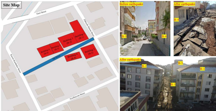
Fig. 10 Site map and earthquake damage on 5th Street
