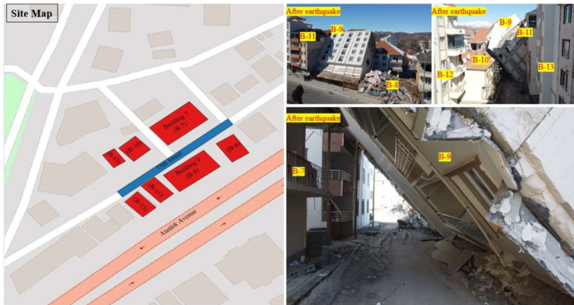
Fig. 11 Site map and earthquake damage on 75th Street
