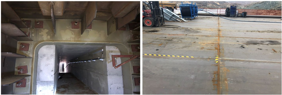
Fig. 11 Views from the steel segments and connections
