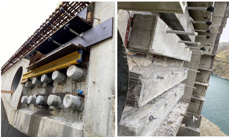
Fig. 9 Views from the anchorage elements at the connection point
