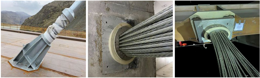
Fig. 10 Views from the cable anchor regions
