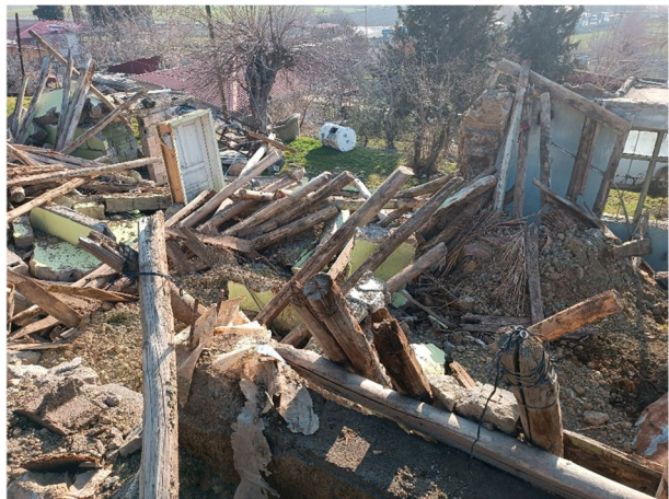
Fig. 31 Heavy damage due to heavy earthen roofs
