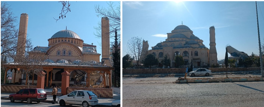
Fig. 36 Examples of minarets damage
