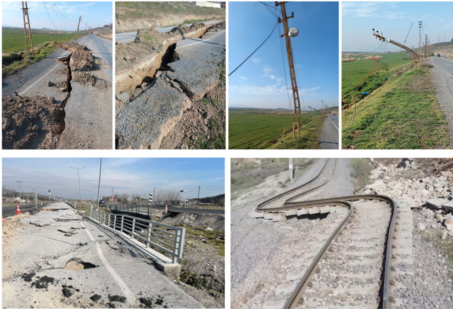
Fig. 11 Damages in transportation and communication facilities after the earthquake (Kahramanmaraş)
