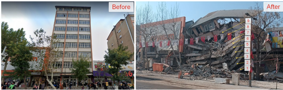
Fig. 14 Sample of pancake total collapse
