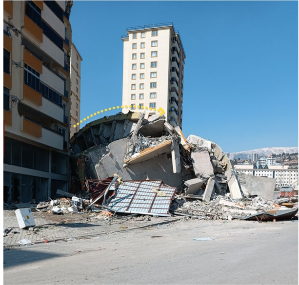
Fig. 18 Lateral collapse (accordion) damages
