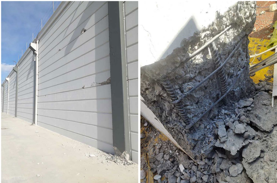
Fig. 34 Plastic hinges formed at the base of the column
